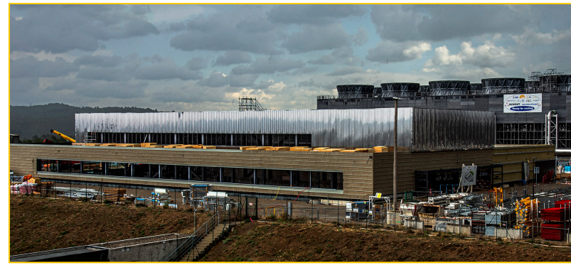
IO access to Control Bldg by Dec 2022
